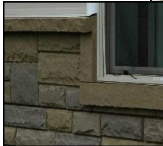
Buff Window and Door Trim installed on sill and sides with Ledger for wainscoting
